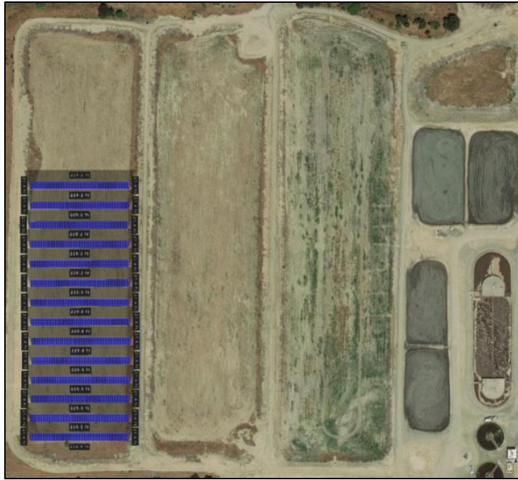
Figure 12: Solar Site for RES-BCT program located at Waste Water Treatment Plant
