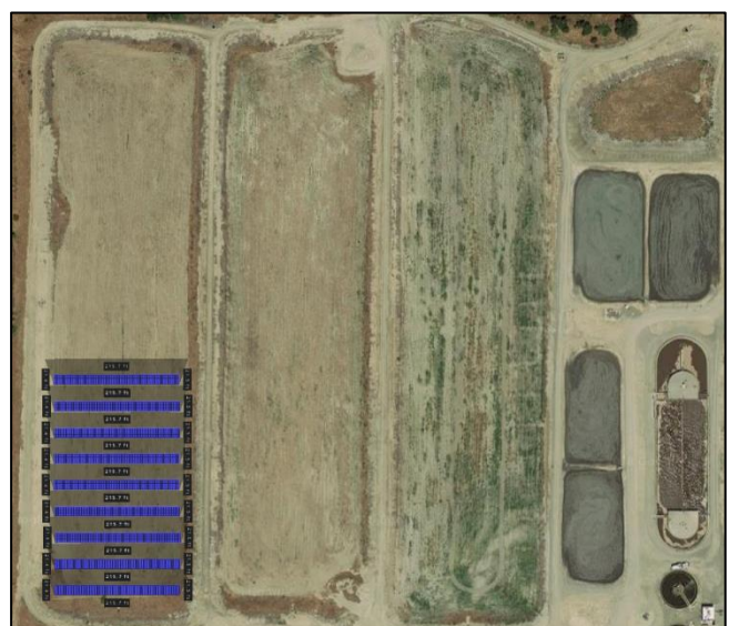
Figure 10: Waste Water Treatment Plant
